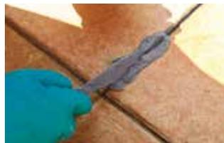
Cracks and discontinuities highlighted by the level of cleanliness must be carefully filled with the special waterproof **STUCCO BALCONY**, including in correspondence with the skirting boards and doorways. Any moveable joints must be treated with **PROTECH FLEX**, the specific polyurethane sealant in an extrudable cartridge with elevated elasticity.
