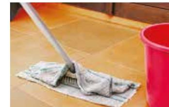
One hour after application, remove any product residue and build-up on the surface of the flooring using a rag with nitro diluent. The transparent non-film waterproofing with high water-repellent power will thus be complete.
